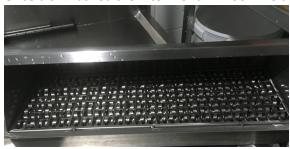
5) With the filters out do a visual inspection inside the exhaust plenum for any grease and fat and wipe remove with a cloth and the approved chemical
