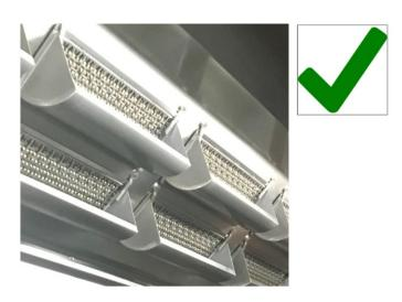
2) To remove the filters 1<sup>st</sup> release the clips that hold them in
