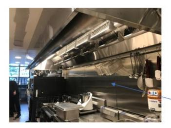
9) Remove any fat and grease from the inside of the hood and clean the front of the bottom of the Makeup air box and the face
