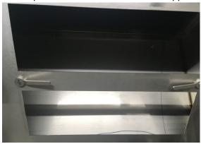
6) Replace the filters – Note there are 2ea pins on the bottom of the filter (you can see them clearly in the image below) – it's critical that you insert the filter angled slightly back towards you, push it in the whole way in then straighten and pull down to ensure that the 2ea pins engage behind the filter mounting panel
